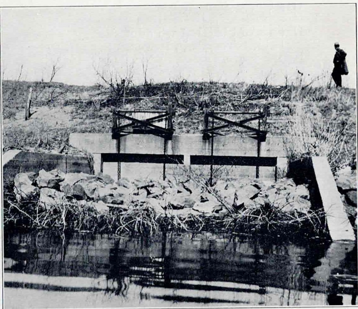
The Delta Gates Closed and the Entrance Filled with Brush and Rock, to Prevent Their Being Opened, Shutting Out the Fish from This Vast Spawning Ground
