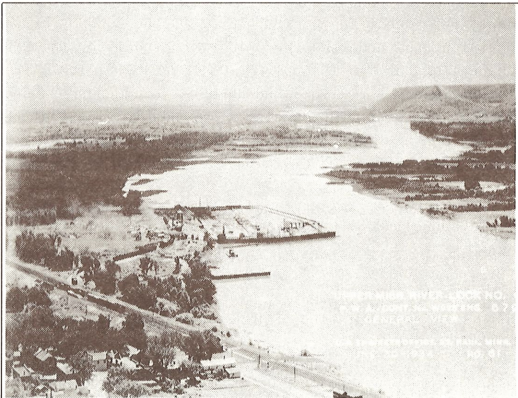
Figure 2 - The Mississippi River at Trempealeau in 1934 showing the temporary coffer dam enclosing the site of Lock Number Six. Looking downstream, Wisconsin shore on the left, Minnesota shore on the right. June, 1934. Corps of Engineers photo.
